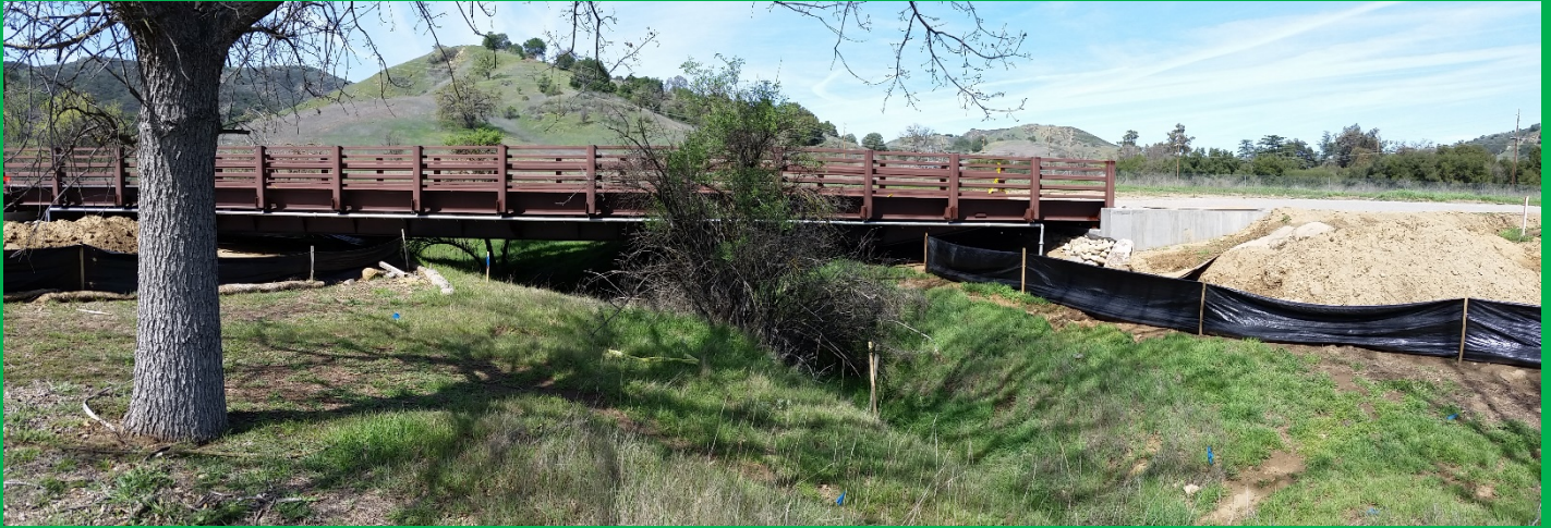
Example of a Prefabricated Bridge within Malibu Creek State Park
