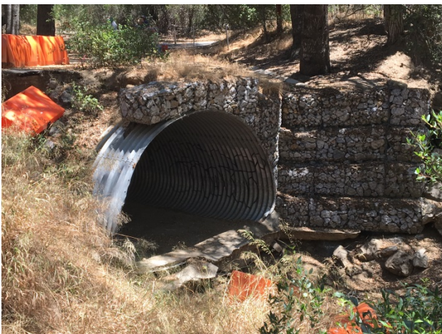
Existing culvert with washed out gabions
