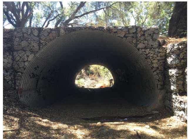
Looking downstream through existing culvert
